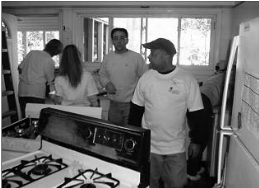
The kitchen received new appliances and much needed repairs.
